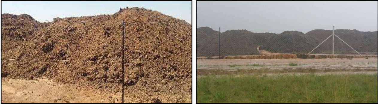
Figure 1: Unprotected Topsoil Stockpiles (before rain on left and during the rain on right)
